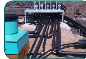
Durapipe PLX is a complete range of dedicated fusion-welded pipework systems for the safe transfer of liquid fuels and their vapours. Suitable for use with leaded, unleaded petroleum, including ethanol rich alternative fuels (E85), diesel, bio-diesel and fuel oils.
